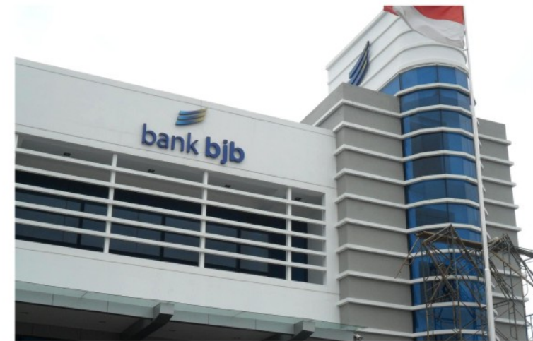
Bank Jabar Banten - Banten, Pile
