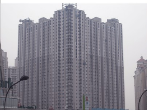
RMG - Jakarta, Facade
