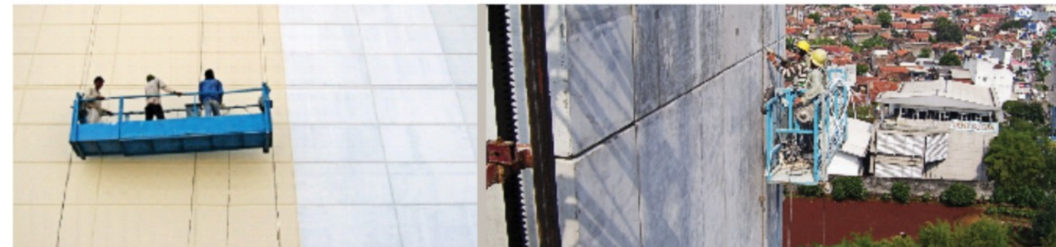
Pemasangan Joint Sealant
